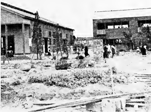
New buildings under construction at Girls' School, Hiroshima
